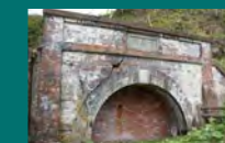
Tenryu Mine Entrance (registered national tangible cultural property)
